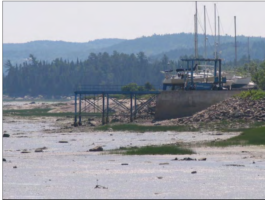
Figure 9. Occupation des infrastructures, Centre Nautique Saint-Martin.
