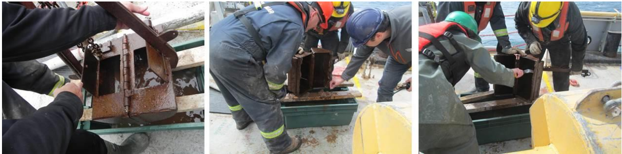
Figure 19. COR1503-BV04 and -BV05 pictures.
