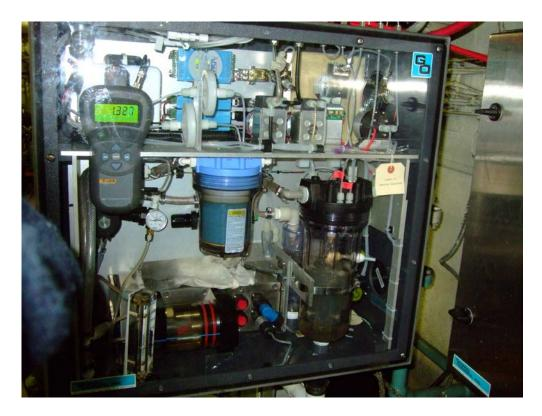
Figure 2.3. The underway system located in the engine room of the Amundsen.
