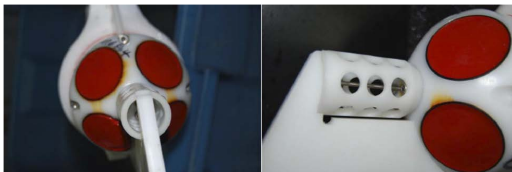
Figure 5.16. Photos of corrosion on DVS 750 transducer heads for Mooring F-09.
