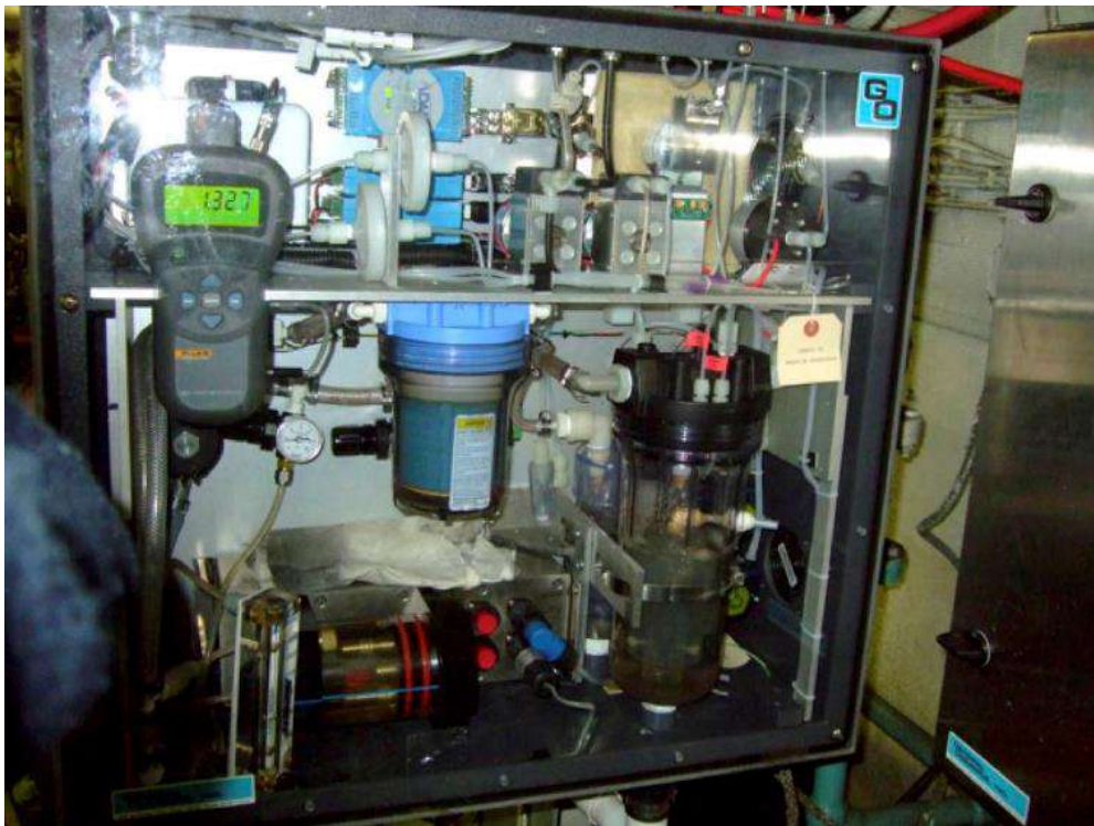
Figure 1-3 The underway system located in the engine room of the Amundsen.
